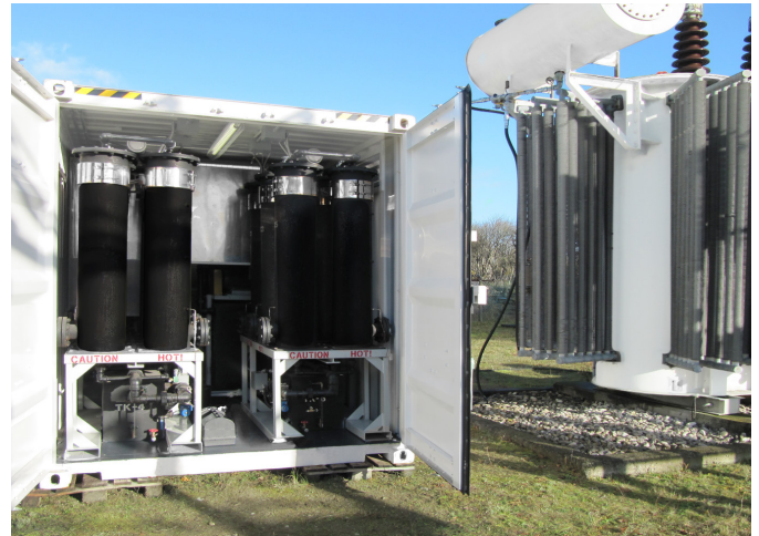
Container Mounted Oil Regeneration System
