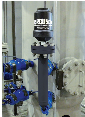
Tri-Magnet level switch and float chamber
